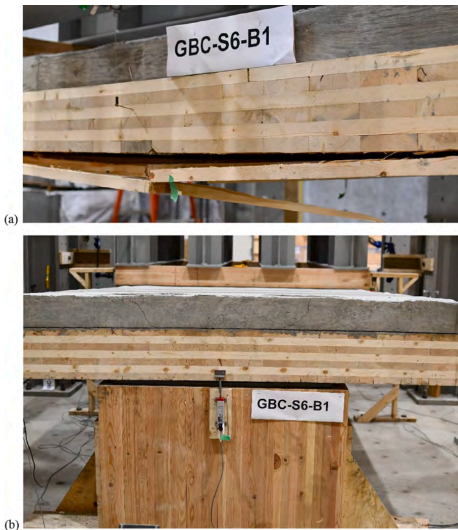
Fig. 11. (a) Typical bending failure in full-scale TCC floors; (b) warping (upward deflection) at support.
